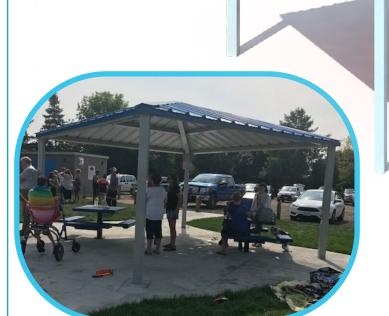
Nirbo Shade Structures are made of A500 Grade B Steel. Steel Structure is hot dip galvanized and powder coated.
